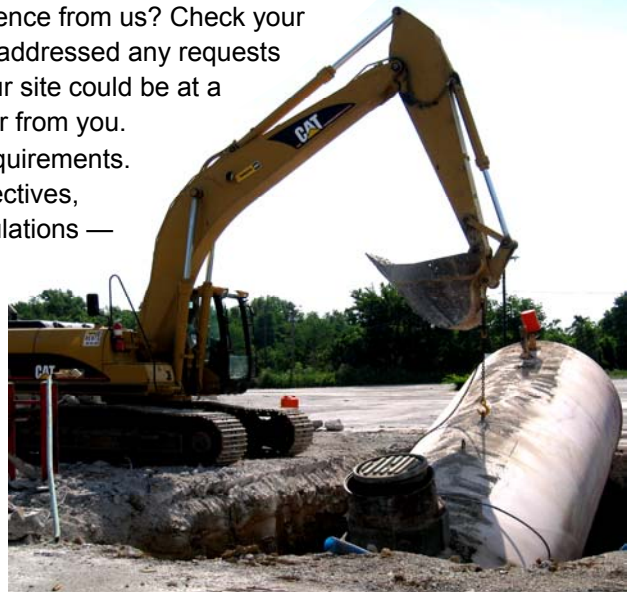
This UST removal was photographed by Trent Garrison, geologist of the USTB Corrective Action Section.
